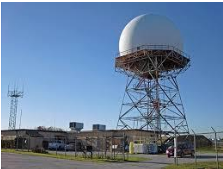
Common Air route Surveillance Radar
